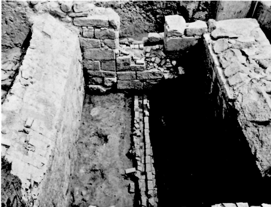
24 2E12. General view of the east end of the British Casemate, showing the abutting below the window, the brick drain, the spring of the arch on the north and south walls. Camera facing east. No scale (2E-181 B).
