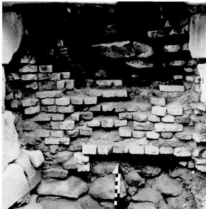
33 2E12. View of the back wall of the fireplace at the east end of the casemate, showing brick wall and rubble wall. Camera facing south. 1 ft. scale vertical (2E-3152 X).
