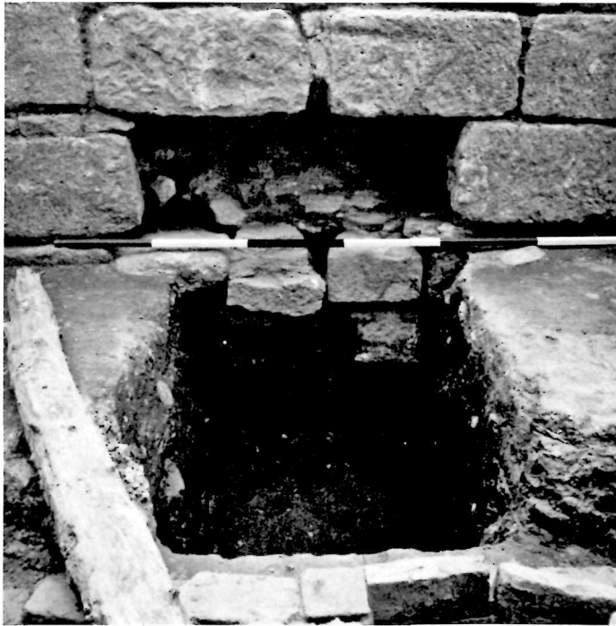
23 2E12Q6. Post excavation shot showing the open space in lower right corner of excavation which is the inlet of drain No. 1, and the difference in construction between the upper and lower parts of the south wall of the casemate. Camera facing south. 6 ft. scale aligned east-west (2E-2062 X).
